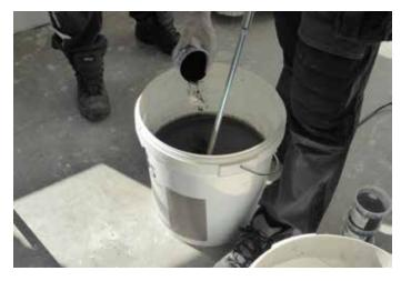
ventilated. Before applying FloorColouring levelling compound, the subfloor must always be primed with 044 Europrimer Multi. This ensures optimal adhesion and prevents the formation of air pockets in the levelling layer.
